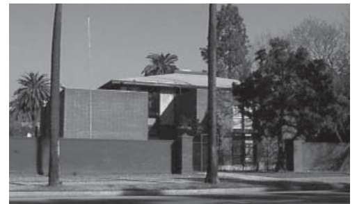
The ONE Archives, the largest archive of LGBTQ materials in the world, is located in an award-winning Modernist former residence built as a fraternity in 1965-1966.
