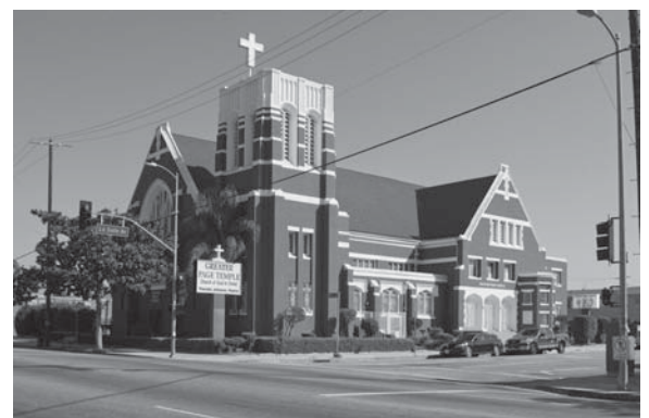
Engine House No. 18 and the Greater Page Temple are among landmark properties in the Charles Victor Hall Tract.
