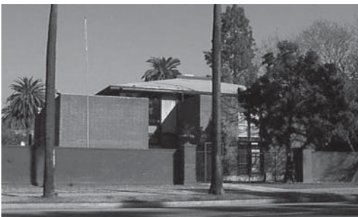
The ONE Archives is located in a Modernist former residence built as a fraternity
