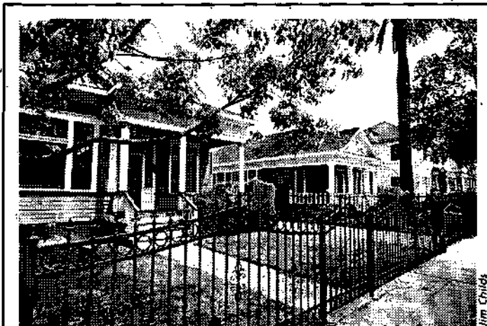
These two houses were rescued from a development in Pico Union, moved by Kristin Belko to 23rd west of Hoover, restored, and sold to private homeowners.
