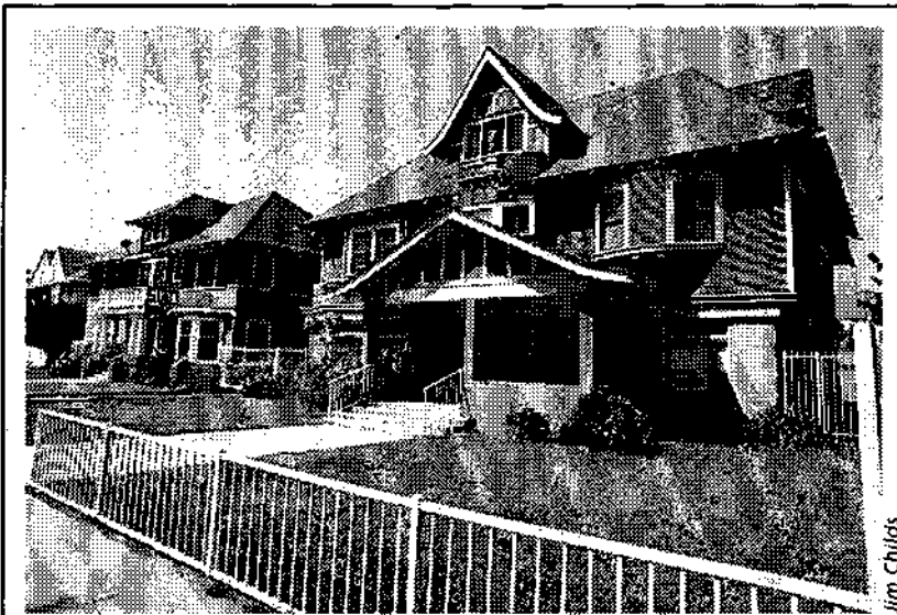
The Community Redevelopment Agency and the Roger Williams Baptist Church relocated three homes on Menlo to new sites, also on Menlo, and converted the structures to senior congregate housing.
